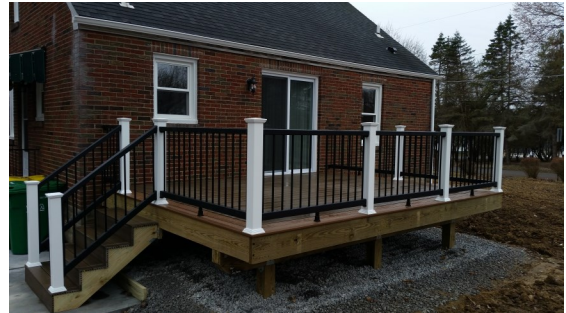
New Deck Gregden Road
