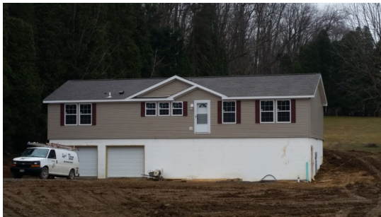
New Single Family Dwelling Dutchtown Road
