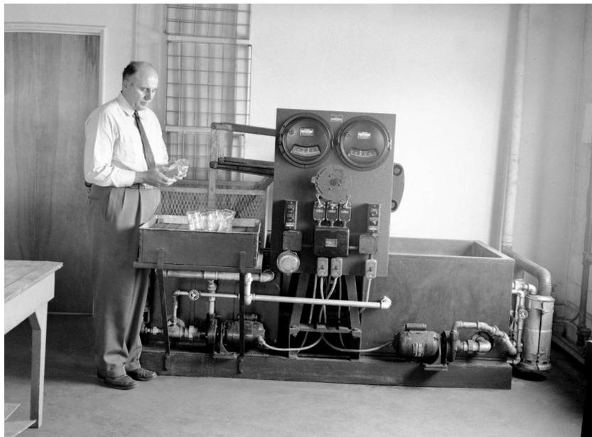
Fig 8: Dr. L. Ghering with an original thermal shock machine. This is the invention that made Preston's career. Using controlled temperatures, bottles (in carrier, left) were immersed in hot water for selected times then moved to a cold water tank (right) and timed until they fractured, determining if they were suitable for the intended use. The modern version is digital. The thermal shock technology is still in use worldwide.
